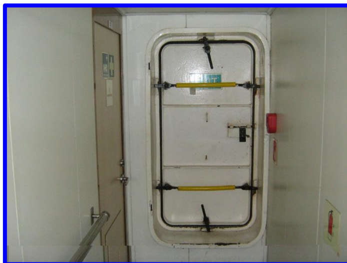
Watertight door effectively secured
