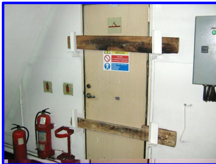
As above – a further deterrent to access should the lock be breached (metal is preferred to wood)
