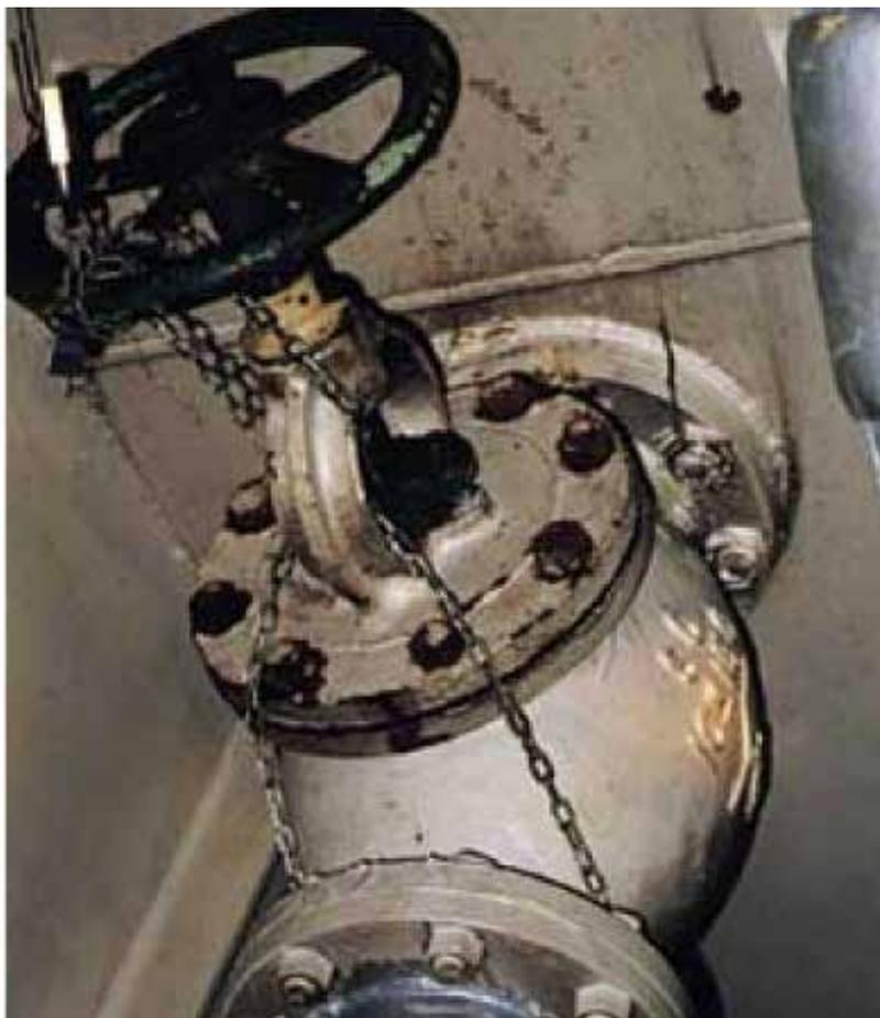
Overboard valve for main bilge/ballast line. The hand wheel has been fitted with a chain and padlock at the request of the port authorities. This is not a good practice as the vessel's bilge pumping system is no longer readily operational.
